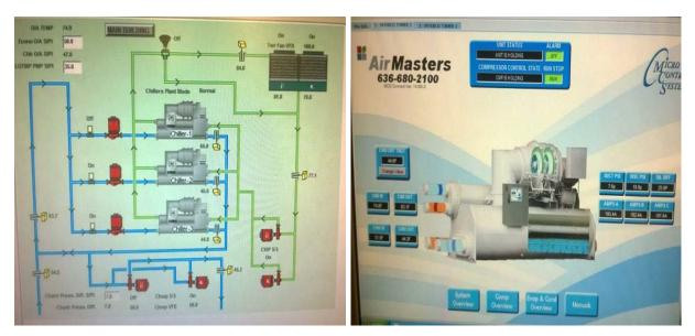
The condenser water reset temperature control, further reduces the lift of the chiller thereby favorably impacting chiller operation and efficiency.
