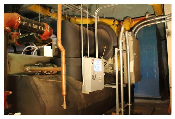
Image 1: Building maintenance personnel can easily monitor and control chiller operation from the touch screen using graphic icons and simple commands
